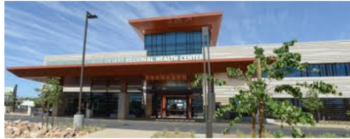
The hub that serves the Antelope Valley exurb is located within the High Desert Regional Medical Center. Photo: L.A. County
